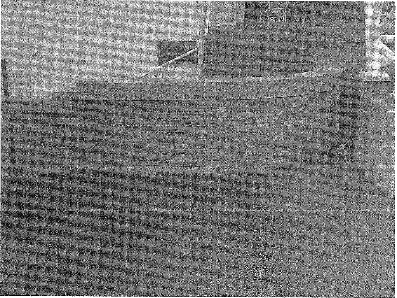
Brick Wall on the East Side of Bandshell Stage
