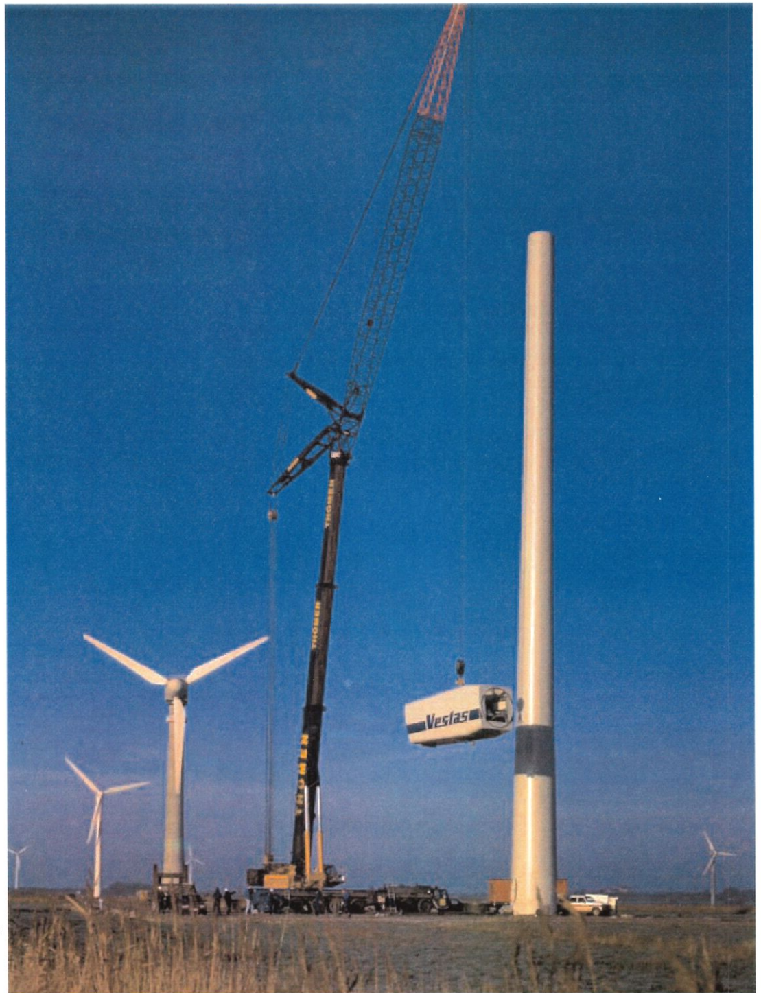
A Vestas 1.5 MW turbine under construction. The "nacelle," or generator is being lifted by crane to the top of the turbine.
