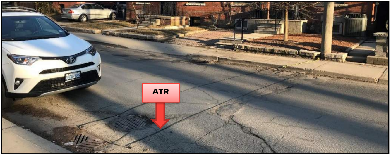
Figure 2.4 ATR Field Installation
