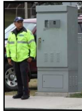
Figure 3.1 Example of Police Officer Operating a Traffic Control Box (Google Street View)
