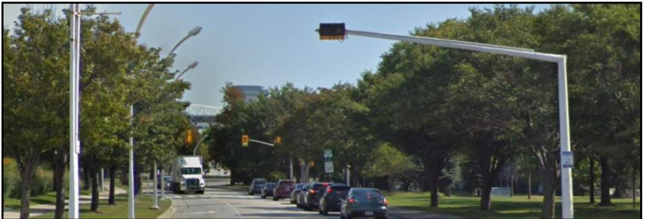
Figure 3.5 Existing Non Functional Reversible Traffic Signal on British Columbia Road (Eastbound) - Google Street View
