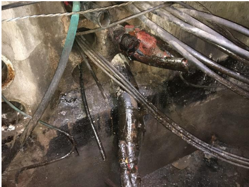
Oily residue observed in Manhole #120
