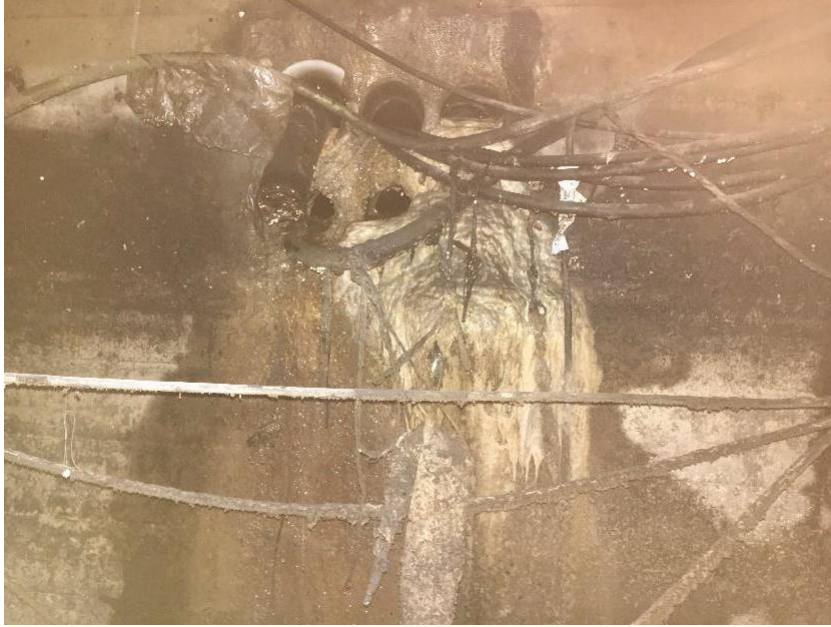
Excessive grime observed in Manhole #130B
