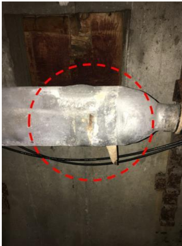
Splice anomaly observed in Manhole #202
