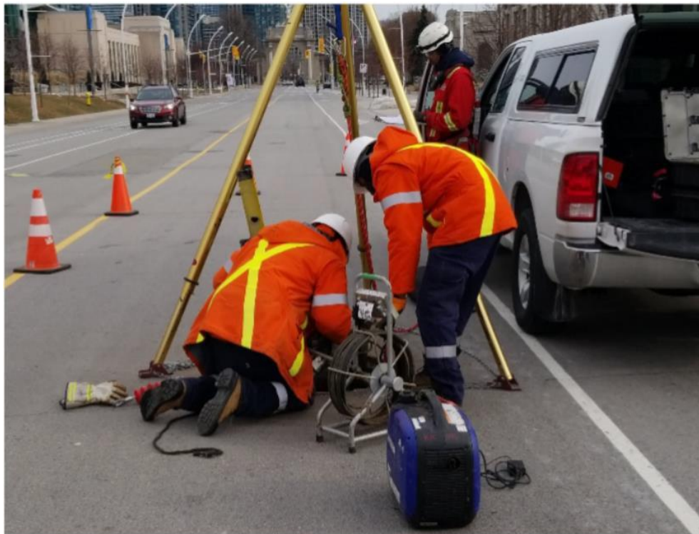
Visual inspection being conducted using an endoscopic camera in Manhole #120
