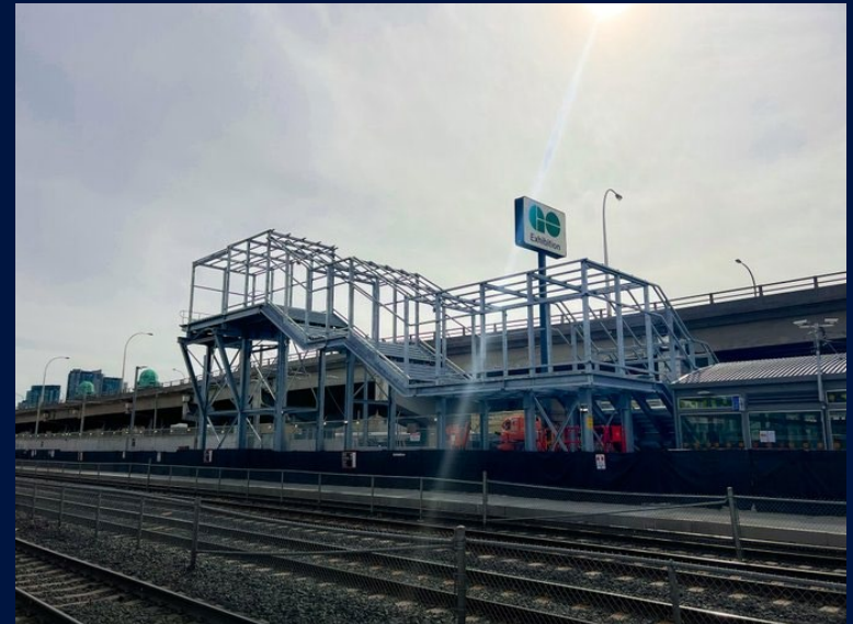
New temporary pedestrian bridge taking shape
