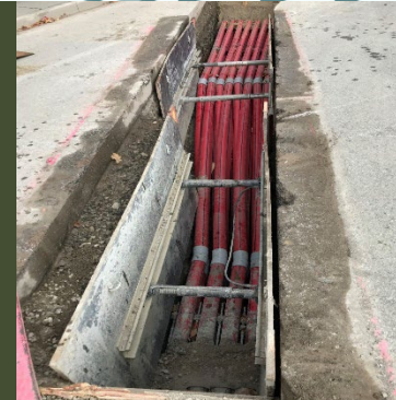
Electrical Duct Bank
